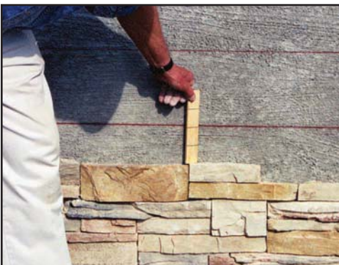
Using a measuring stick
